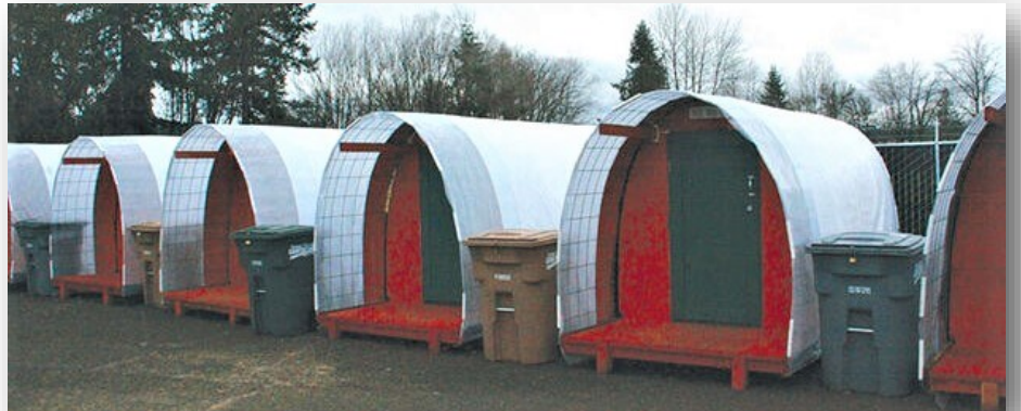
Huts built by Sweet Home High School students and volunteers at the new homeless shelter in Sweet Home. The shelter is on property donated by Linn County. Photo courtesy The New Era.
