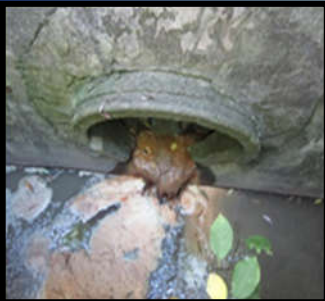
Septic, sewage, and dumping or disposal of liquids or materials other than stormwater.
