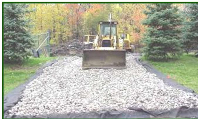
***-Construction Entrance*** located where traffic leaves a construction site. As vehicles drive over the gravel, mud, and sediment are collected from the vehicles' wheels and offsite transport of sediment is reduced.
