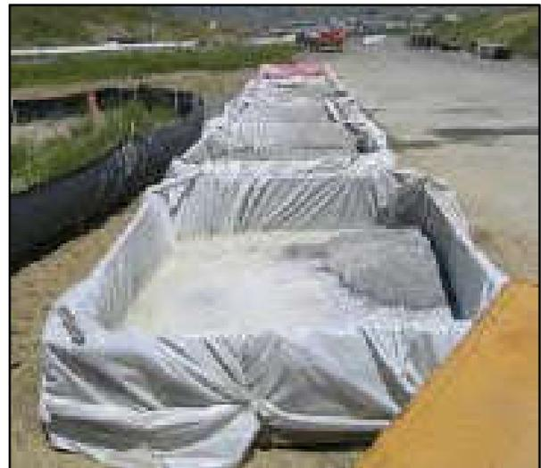
**Image 30.** Plastic Sheetting Lined Concrete Washout Basin
