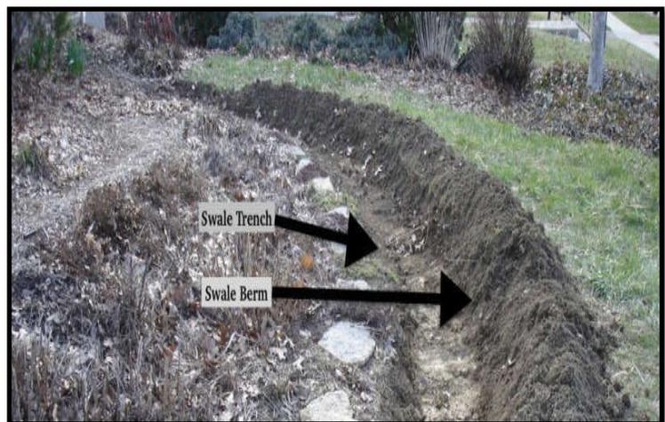
**Image 12.** Soil Dike with Swale
