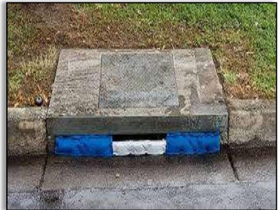
**Image 22.** Curb Inlet Sediment Dam
