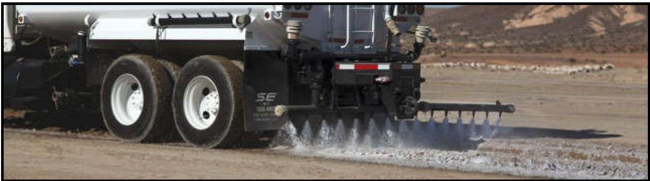
**Image 3.** Soil Binder Being Hydraulically Applied to Bare Soil
