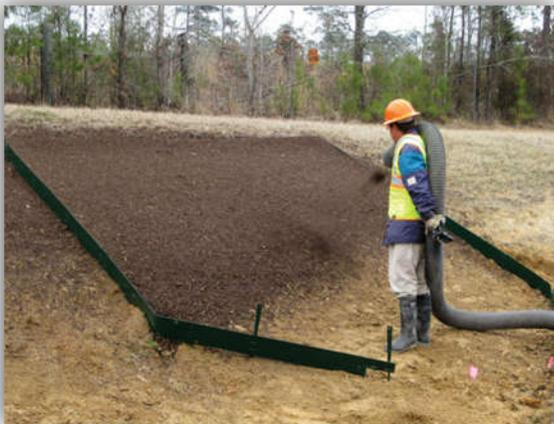
It is typically applied to slopes with pneumatic blower trucks (Image 7). Compost erosion control blankets act similarly to mulch products but provide organic nutrients that promote vegetation growth, even in areas where germination, moisture management and irrigation could be challenging.
