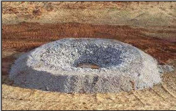
**Image 17.** Aggregate Inlet Protection
