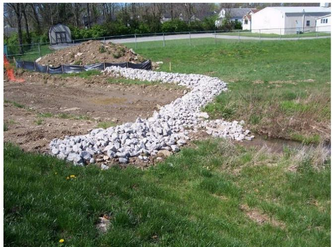
**Image 26.** Aggregate Filter Berm
