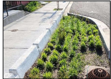
Image 8. Sidewalk Drainage Notch
